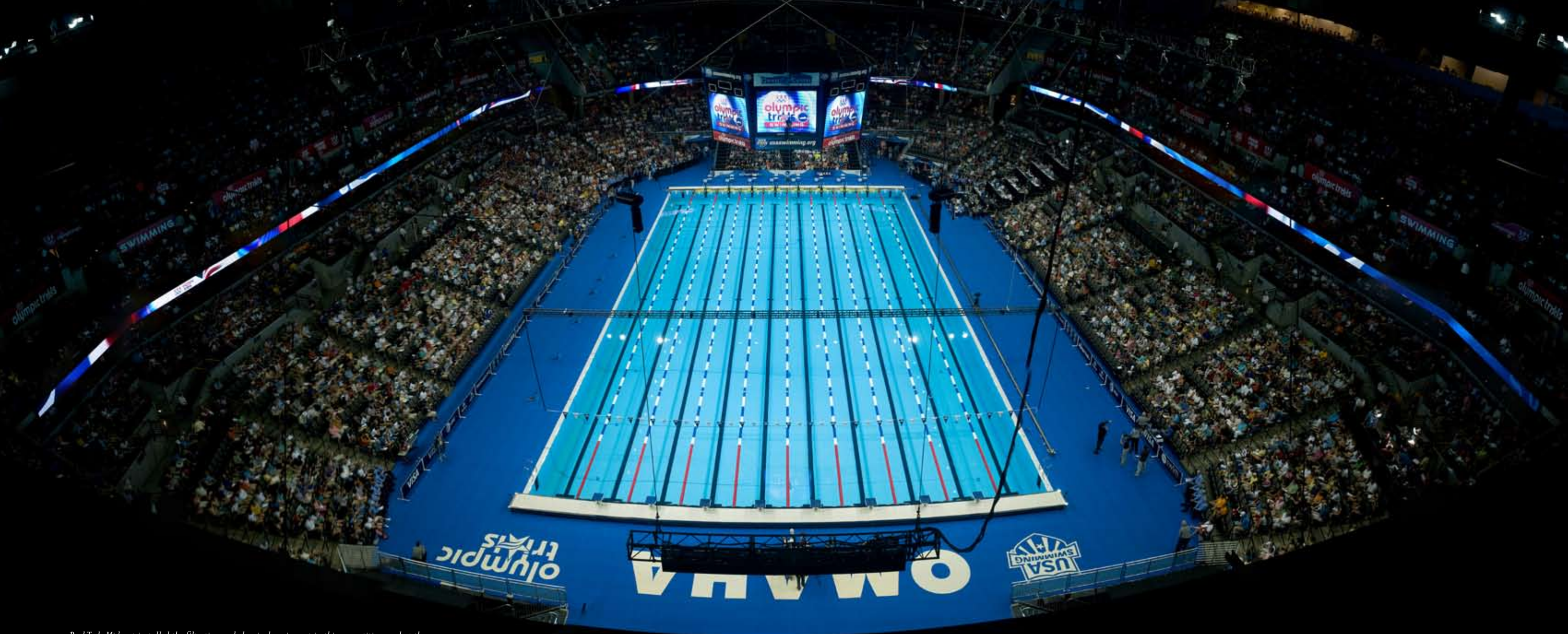
Pool Tech Midwest installed the filtration and chemical equipment in this competition pool at the Quest Center in Omaha, NE, which was used for the 2008 Olympic time trials.
